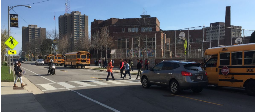
Figure 13-2 Marked Midblock Crosswalk.
