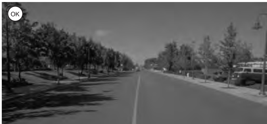
Figure 2-5: In some areas with plenty of off-street parking, collectors are designed for on-street parking with extra space for bicycles. This may result in excessive width and potentially high traffic speeds.
