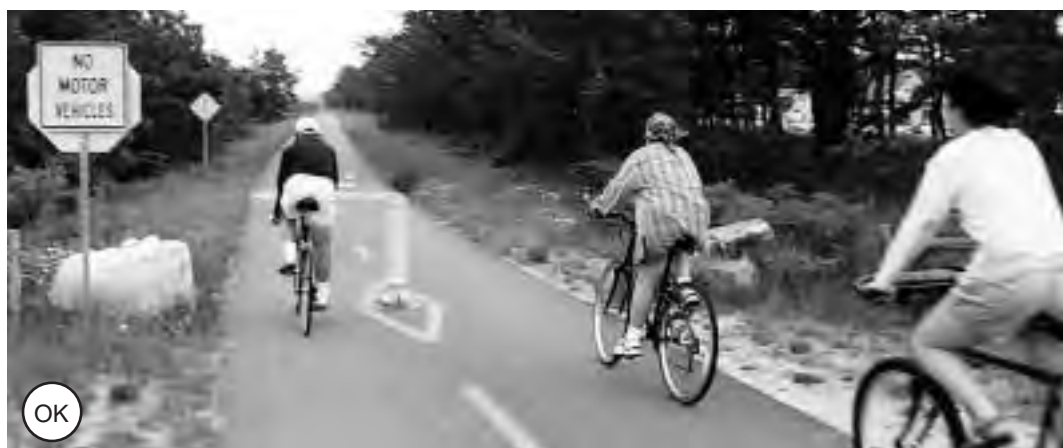
Figure 4-147: The bollard in the middle of this path entrance will not stop motorists from entering. It is, however, highly visible and has the appropriate pavement markings. Still, other elements should be the first choice to discourage encroachment.
