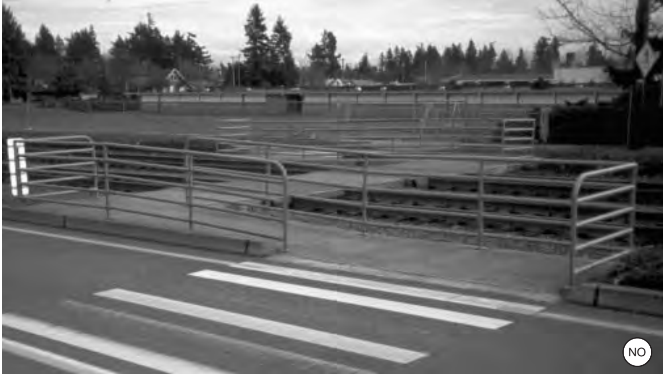
Figure 4-143: A maze intended to discourage motorcyclists. In general, anything that will keep motorcyclists off a path will make use difficult for bicyclists, tricyclists, and wheelchair users.
