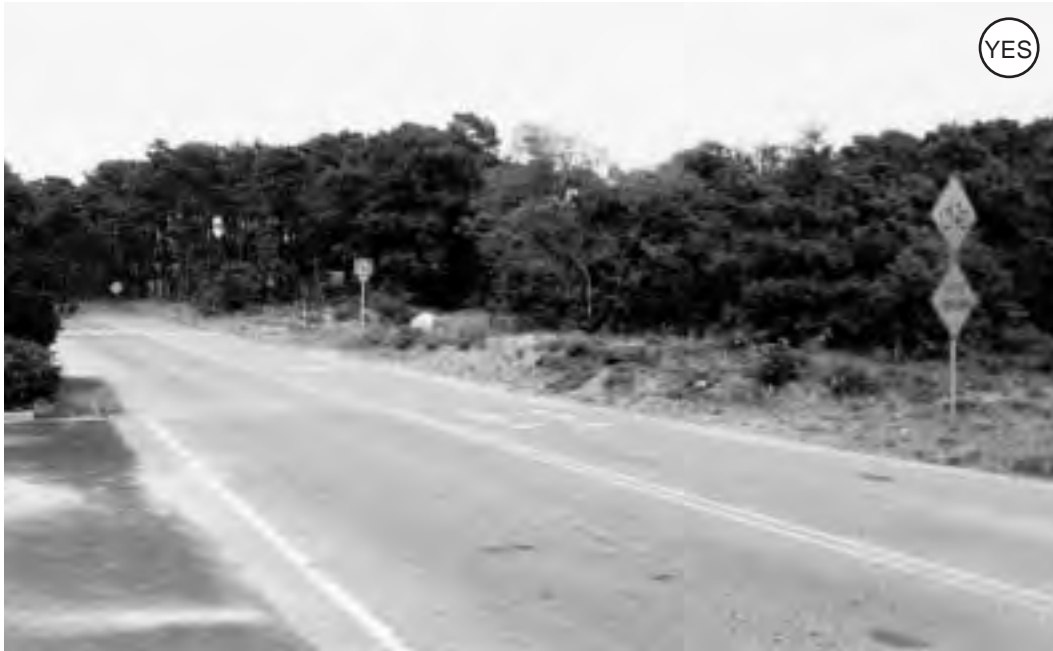
Figure 4-86: A shared-use path crosses a rural low-volume highway. Signing and marking, combined with good sight distance, are the primary requirements.
