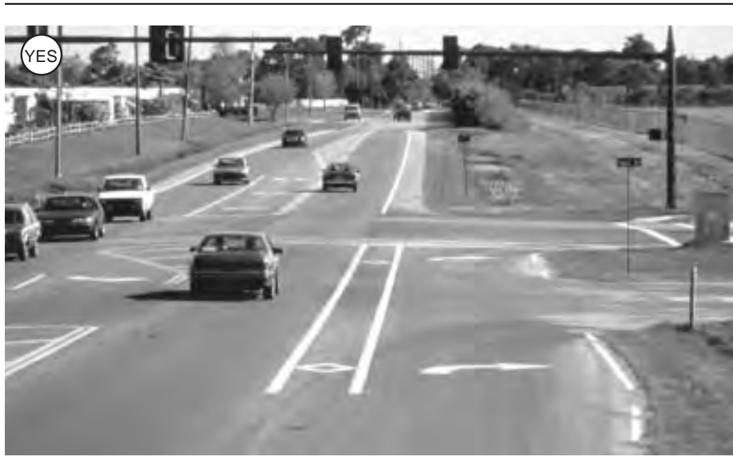
Figure 3-37: This intersection features a bicycle lane to the left of a right-turn lane. Note how it lines up with the bicycle lane on the far side of the intersection.
