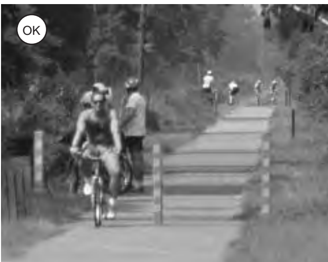
Figure 4-151: If bollards are necessary, they should be reflectorized, positioned in a highly visible location, and separated by 5 ft. (1.5 m).
