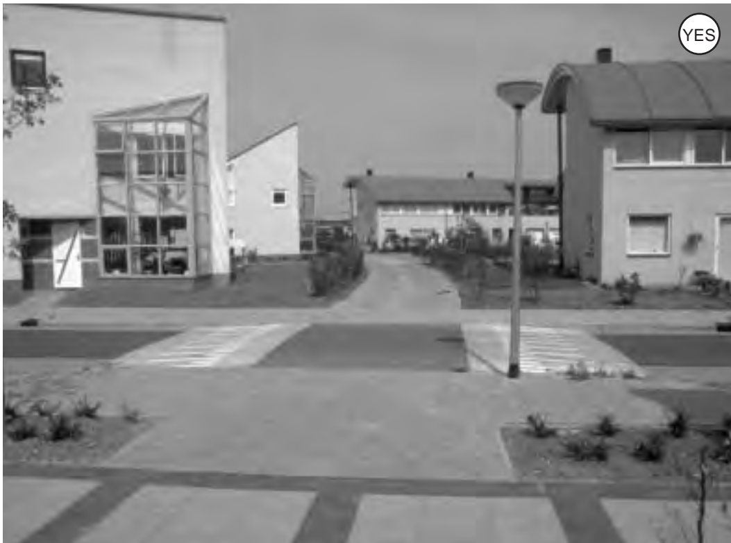
Figure 4-97: A raised path crossing used to slow motorists and give path users priority.
