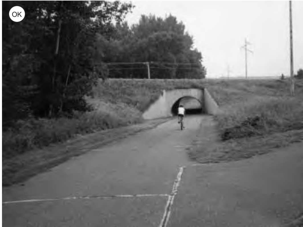
Figure 4-88: A grade separation takes bicyclists under a moderately busy highway. Sightlines are good and the entry and exit grades are slight.
