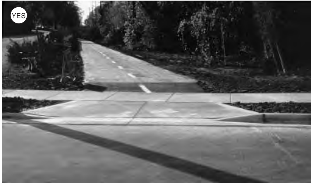
Figure 4-145: Often, nothing special is needed to discourage motorists from using a path.
