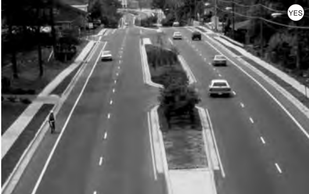
Fig. 3-2: Bicycle lanes should be one-way facilities, carrying traffic in the same direction as the adjacent motor vehicle travel lanes.
