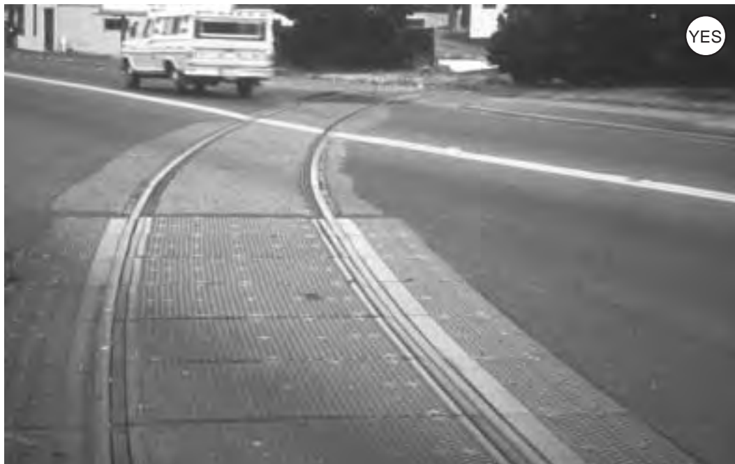
Fig. 2-41: Fillers can completely eliminate the field flangeway gap but must allow for the train wheel in the gauge flangeway.
