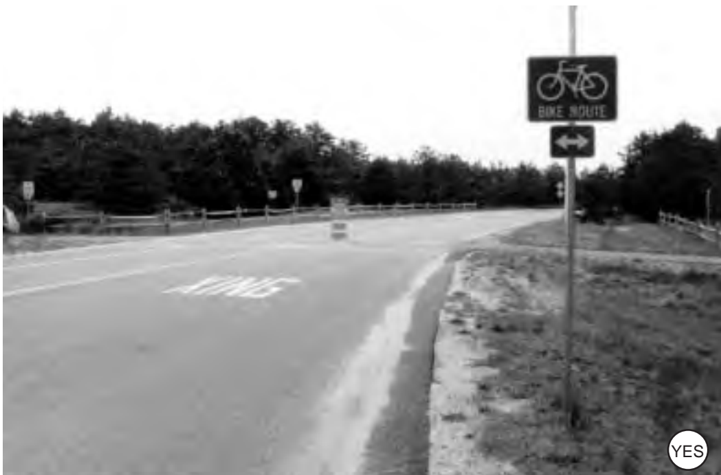
Figure 4-94: This rural crossing has excellent sight distance for both motorists and bicyclists. Signing and marking make it clear what to expect.
