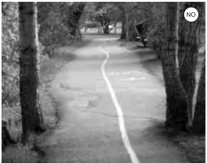
Fig. 4-40: Poor alignment reduces the effective width of this path.
