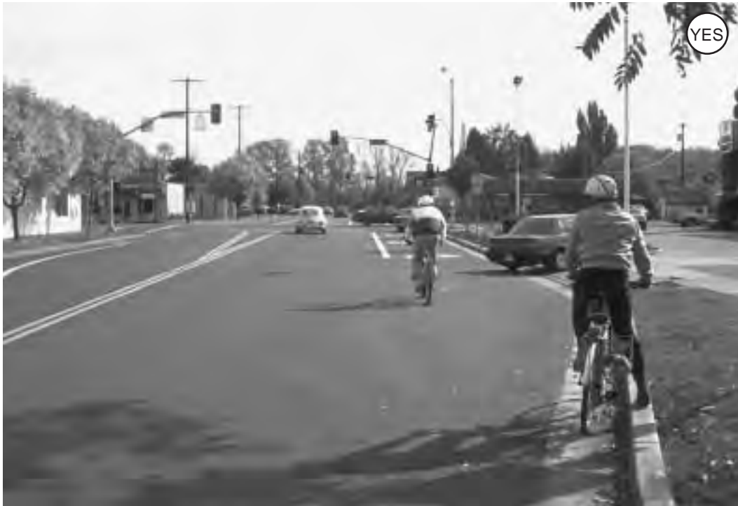
Figure 2-60: At the end of a bridge with wide outside lanes, the extra width should continue in the through lane rather than the right turn lane.
