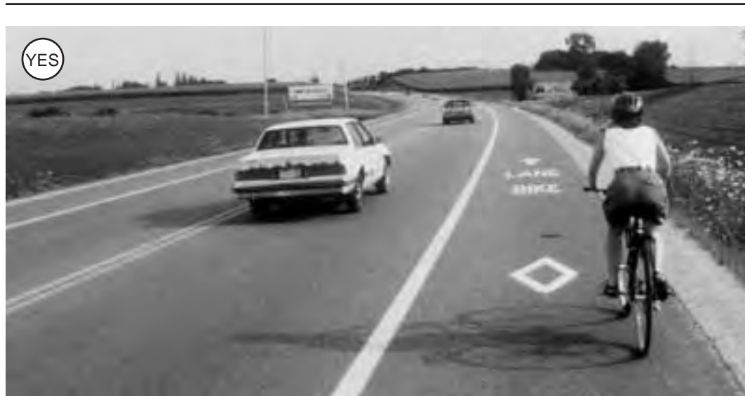
Figure 2-32: Adequate paved shoulders on rural roads provide clearance between bicyclists and passing motorists. In this particular instance, the shoulder is marked as a bike lane, since it links a state park entrance and a state trail.
