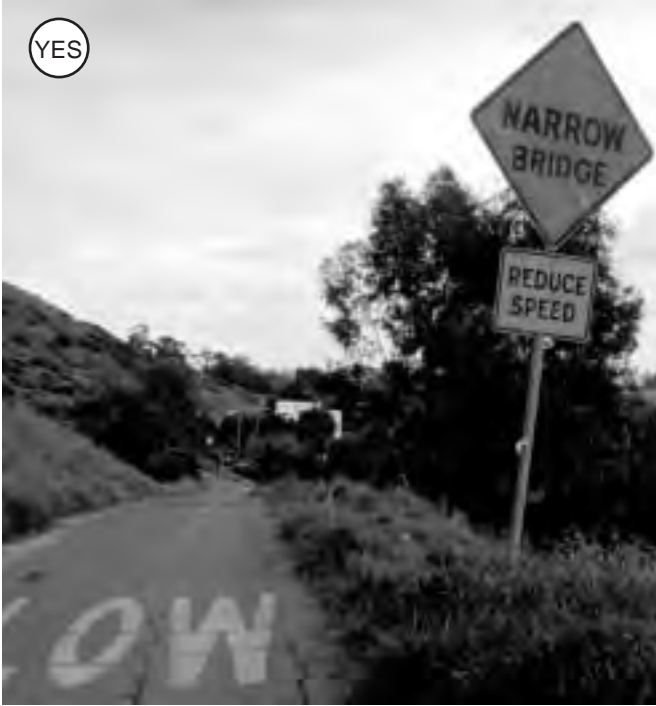
Figure 4-75: Warning signs offset from the path's edge for safety.
