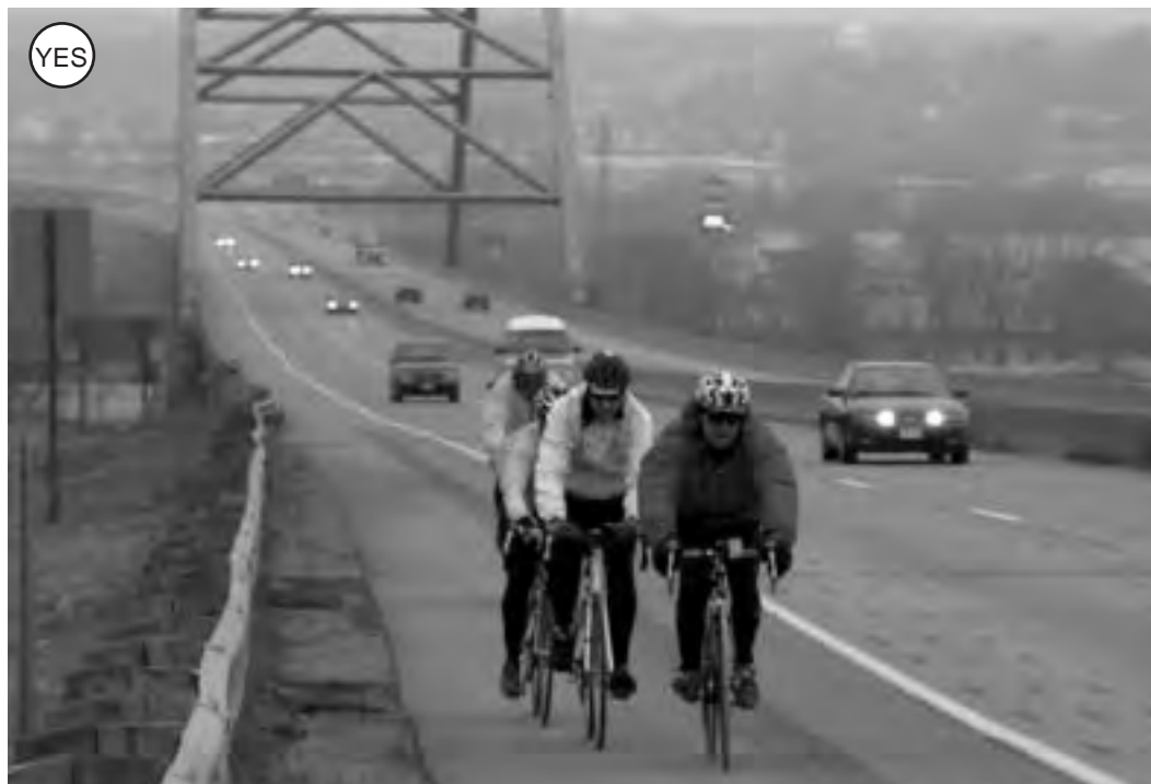
Figure 2-53: Bicyclists using the shoulder of a highway bridge. Note lack of debris and smooth pavement, aspects that bicyclists appreciate.
