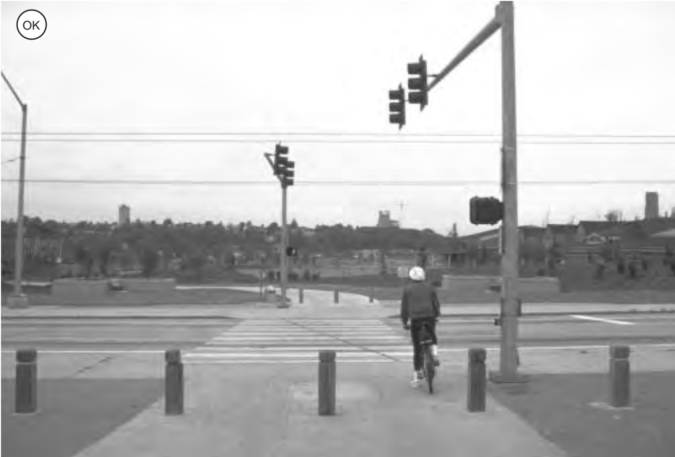
Figure 4-103: An independent signalized crossing for a suburban path. (Note dark, marginally-reflectorized bollards — a hazard, particularly under low light conditions.)
