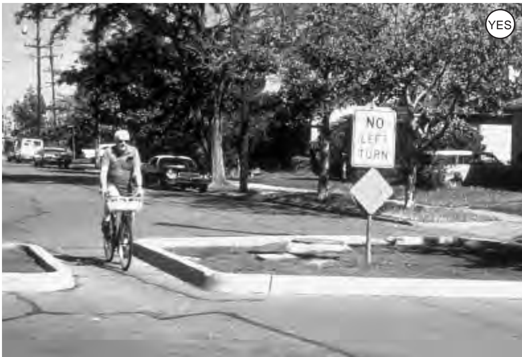
Figure 2-66: This mid-block street closure is part of a “bicycle boulevard,” a through route for bikes that avoids an adjacent busy arterial street.
