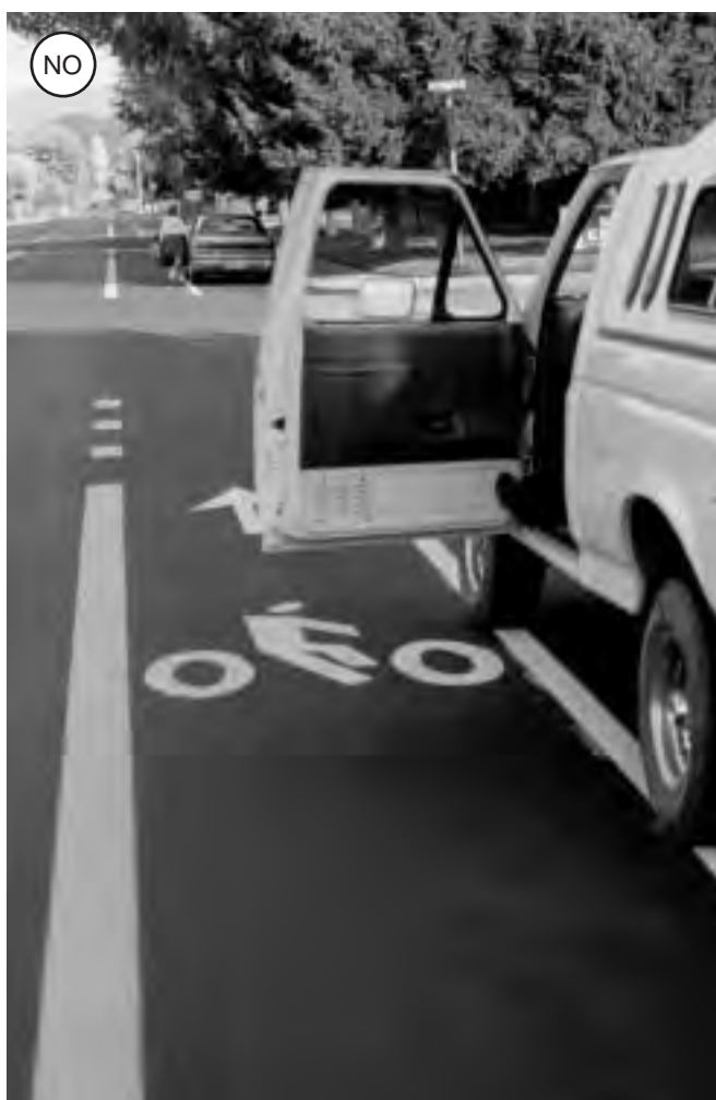
Fig. 3-17: An otherwise adequate bicycle lane next to a very narrow parking lane.
