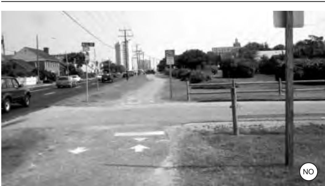
Figure 4-110: Positive features of this crossing are good visibility and proximity to the roadway intersection. Problems include lack of crosswalk marking and confusing right-of-way assignment (bicyclists apparently required to yield to motorists who have a stop sign).
