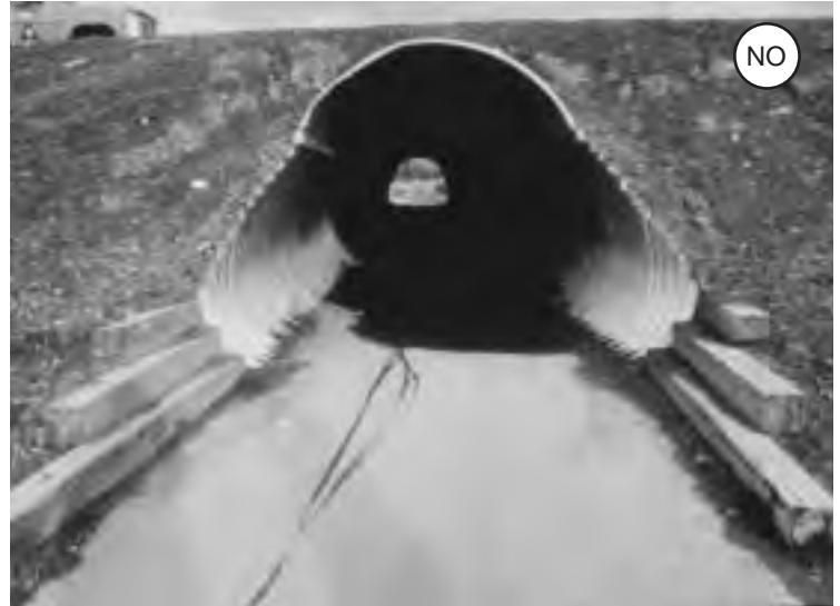
Figure 4-115: A dark, damp, and uninviting underpass. In addition, the path entrance should be flared out to eliminate the path-side hazards.
