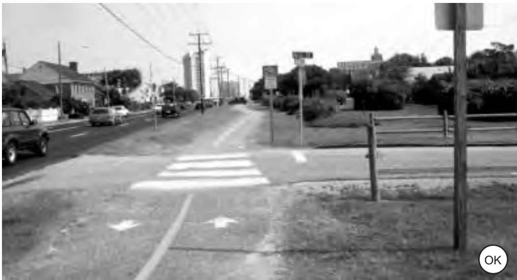
Figure 4-111: Some elements that would help include highlighting the crossing, moving the stop sign and stop bar for the crossroad, as well as adding appropriate warning signs (not shown). Still, motorists will tend to stop in the crosswalk to wait for traffic and the design is far from optimal.
