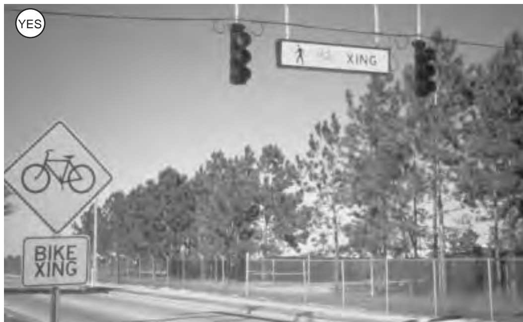
Figure 4-112: Warning devices let motorists know there is a path crossing.
