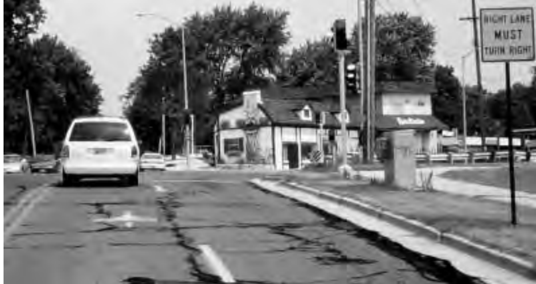
Figure 2-46: Traffic signal systems should be designed with bicyclists in mind. Note bicycle pavement marking for signal loop detector in through lane.
