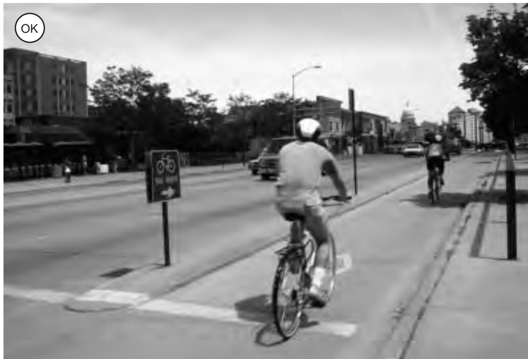
Fig. 3-8: A contra-flow bicycle lane on a one-way street protected by a barrier because of high volumes of opposite-flow motor vehicle traffic. On the far side of the street, there is another bike lane for bicyclists going the same direction as traffic.
