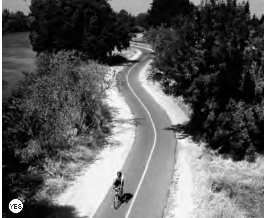
Figure 4-20: An example of a trail with gentle curves, good visibility, and clearances.
