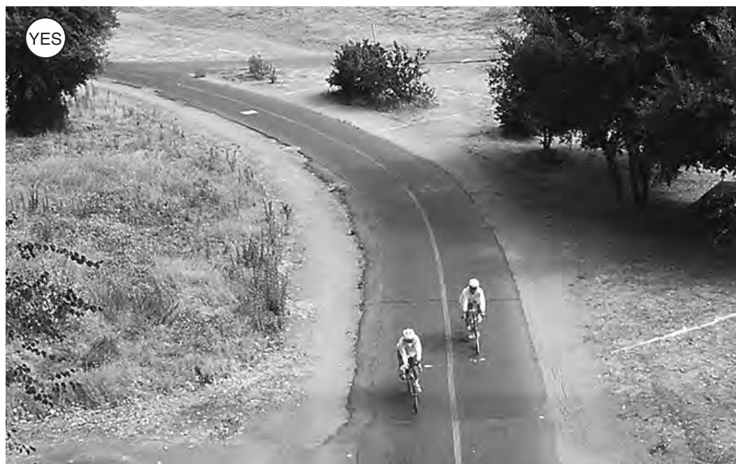
Figure 4-16: Using an adequate design speed means better visibility at curves and a reduced potential for unexpected conflicts.
