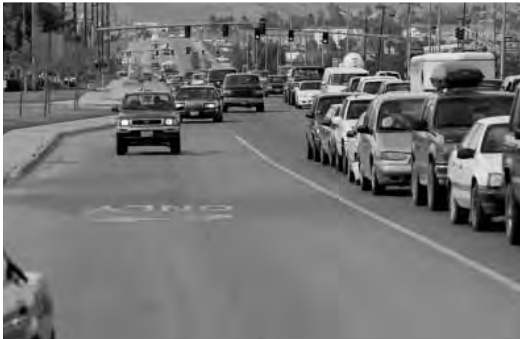
Figure 2-6: A major suburban arterial street with 45mph speeds and high volumes. Many bicyclists would see this as a hostile bicycling environment.
