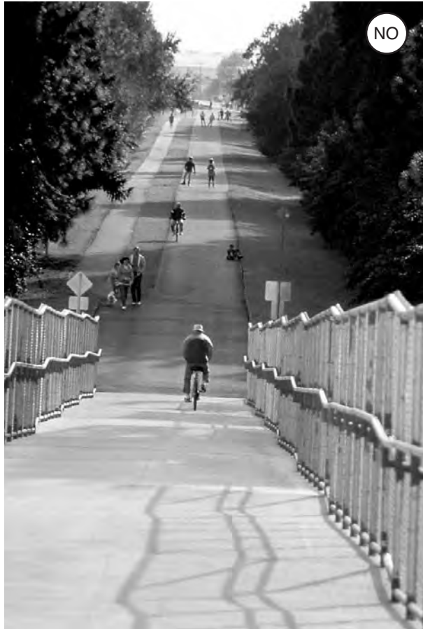
Figure 4-122: While this ramp provides landings and meets ADA slope limits, the overall length and height make it impossible to use for many disabled people.
