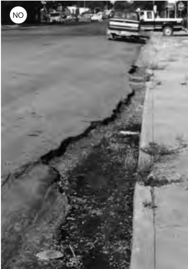
Figure 2-10 (above): Bad pavement edges create hazards for bicyclists.
