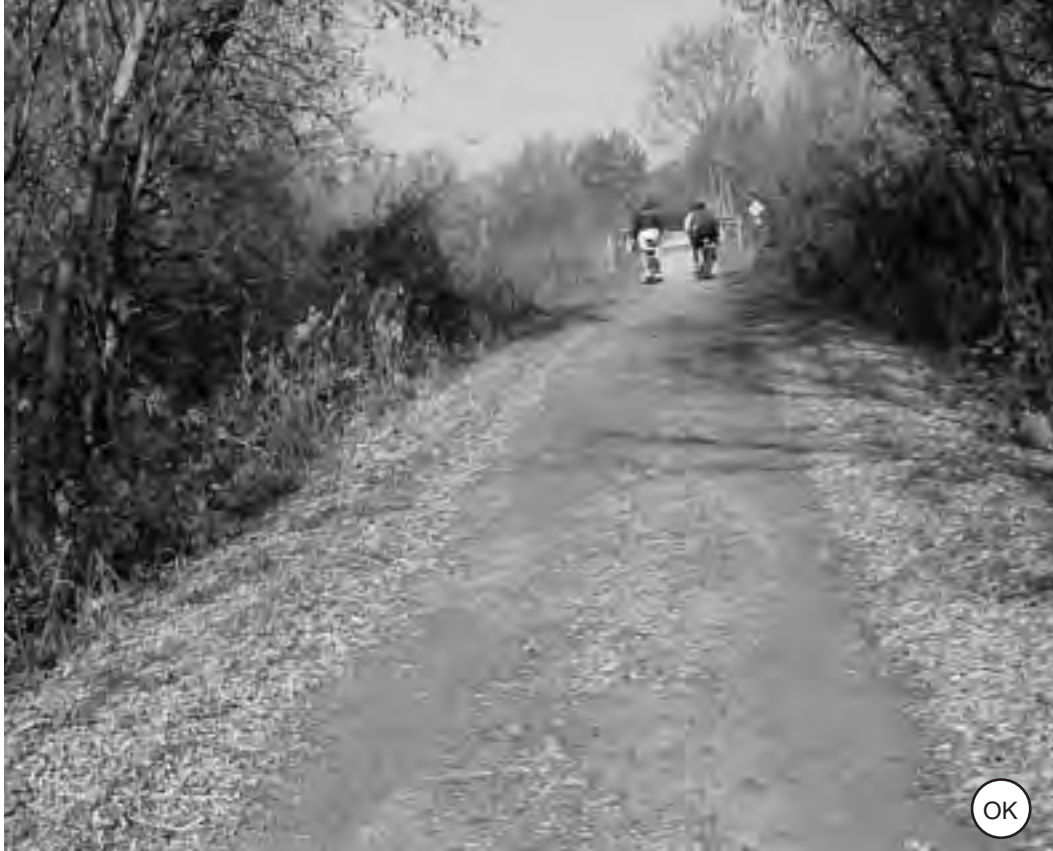
Figure 4-46: A crushed stone path often has a more natural appearance than pavement and is particularly good for trails following abandoned rail lines.
