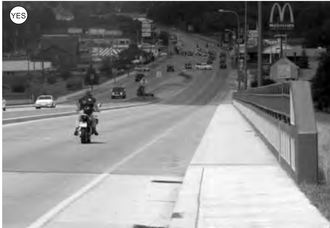
Figure 2-55: A suburban bridge with 5-ft shoulder for bicycles, as well as a sidewalk.
