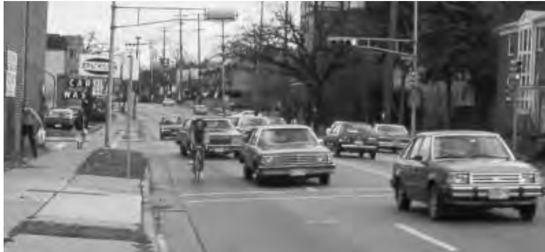
Figure 2-28: On an arterial street with narrow right-hand travel lanes, drivers will either pass bicyclists in close quarters or shift into the adjacent lane to pass.
