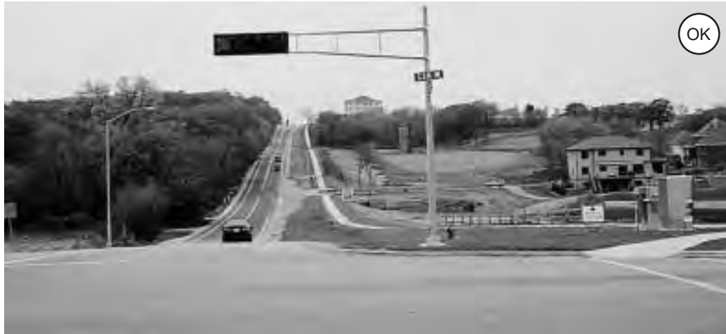
Figure 2-34: Paved shoulders are most helpful in developing areas. In such cases, new land uses typically lead to higher traffic levels, often rendering old rural roads inadequate and hazardous for bicyclists. Note temporary shoulders.
