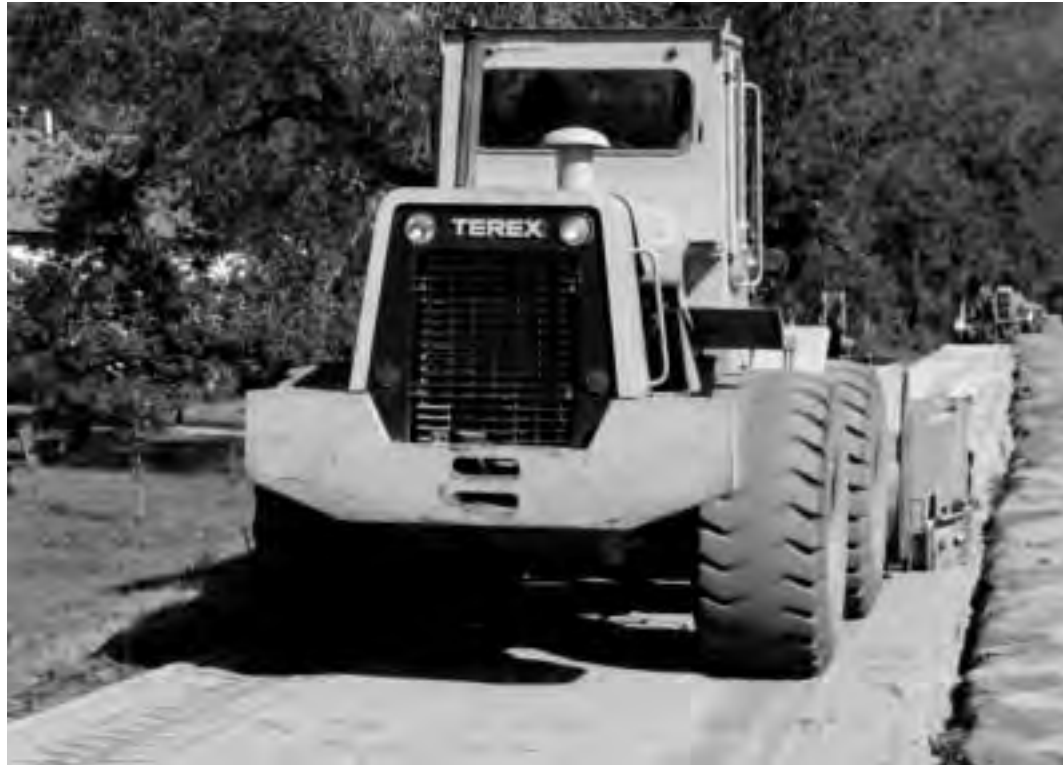
Figure 4-41: Preparing shared- use path subgrade.
