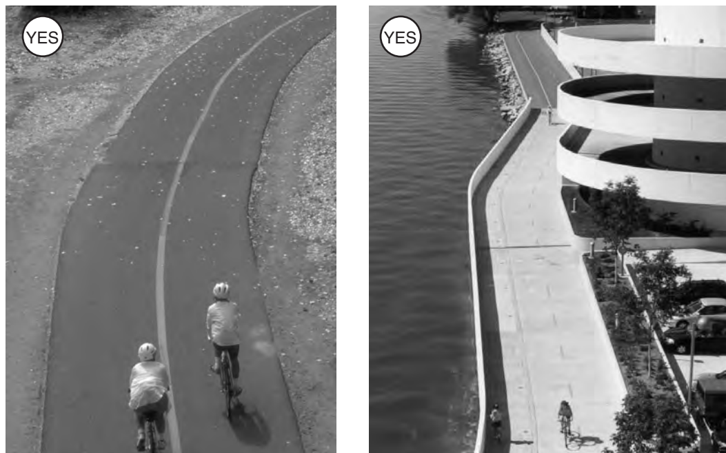
Figure 4-1 (left and right): Shared-use paths often serve as necessary and important extensions to the roadway network.
