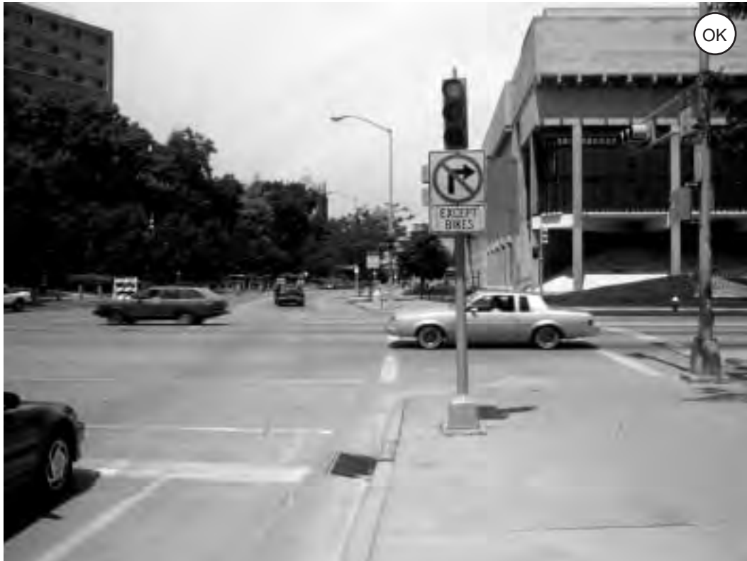
Fig. 3-9: Providing side street signage is an important element in creating a safe contra-flow bicycle lane. Note that the contraflow bike lane street is not signed as a one-way street. Motorists are simply prohibited from turning the wrong way.
