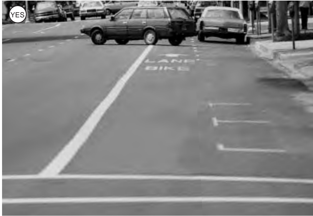
Figure 3-34: Bicycle lane stripes should start at the marked crosswalk or the extension of the adjacent property line.
