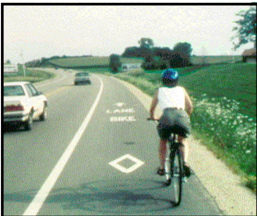
Bike lane shoulder on Hwy 23
