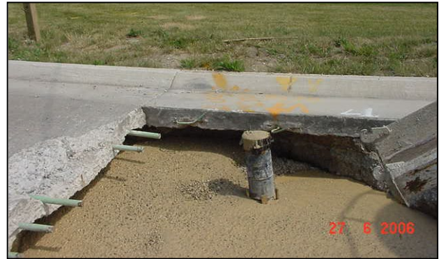
Figure 2: Concrete pavement repair without sawcut. Note top of pavement edge and missing dowel bar. In lower picture, dowel bars in gutter are bent and not ready to accept slurry.
