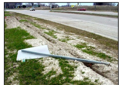
Figure 1: Improper Sign Removal
