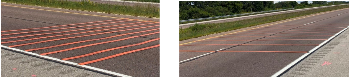
Figure 21.4 Temporary Rumble Strips
