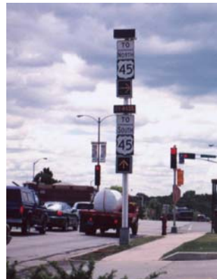
Figure 25.3-4: Alternate Mounting Configuration in Narrow Clearance Areas
