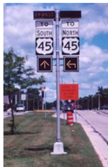
Figure 25.1-1: Typical Dynamic Trailblazer Assembly
