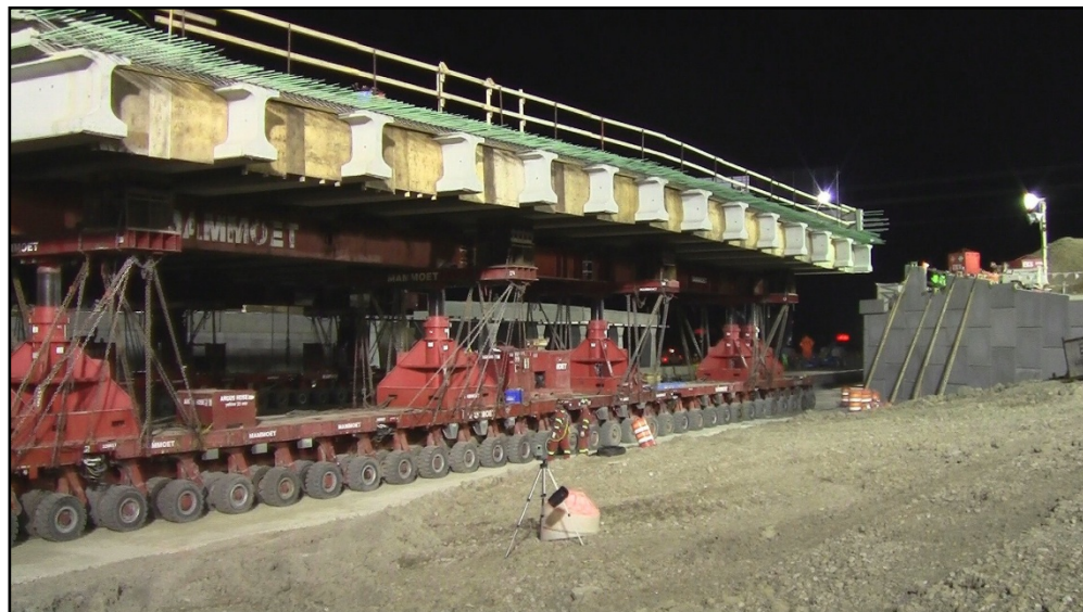
Figure 7.1-7 Self Propelled Modular Transporters Moving a Bridge
