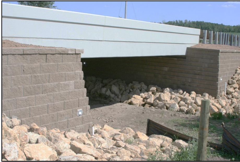
Figure 7.1-4 GRS-IBS Structure
