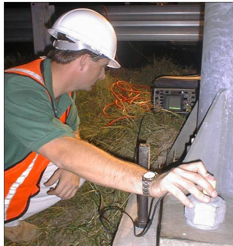
Figure 5.5.2-1: Inspector Conducting UT on a Sign Structure Anchor Bolt.
