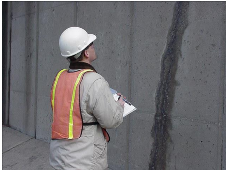
Figure 5.2.1-1: Inspector Conducting Visual Inspection.
