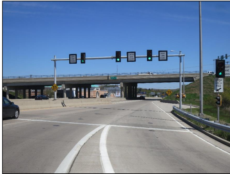
Figure 4.2.3-49: Monotube Sign Structure with Signal Heads Attached to Horizontal and Vertical Members.
