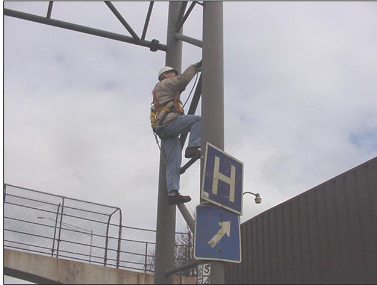
Figure 4.2.2-1: Inspector Climbing an End Support Frame.
