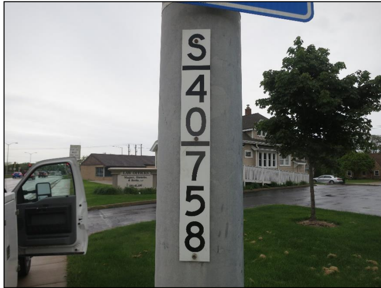
Figure 4.2.4-10: Structure ID Plaque on Column of Sign Mast Arm Structure.
