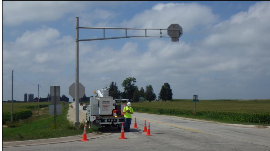
Figure 4.2.1-11: Typical Trombone Arm Sign Support Structure.
