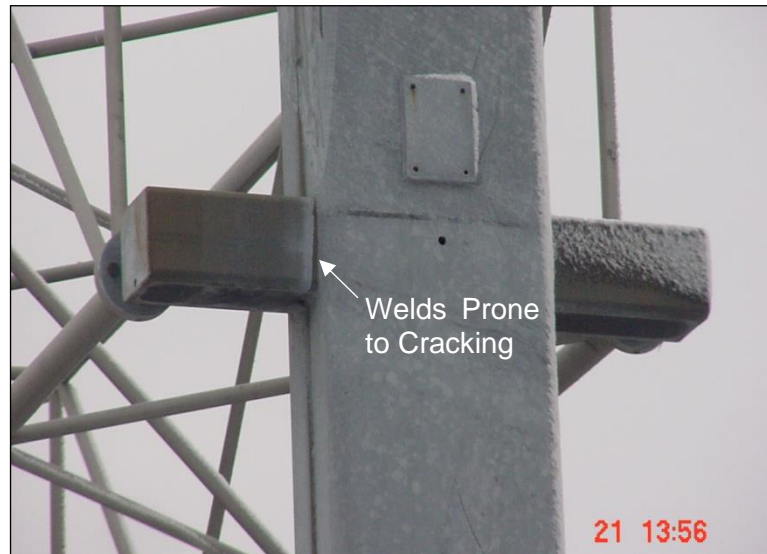
Figure 4.2.3-25: Square Stubs Welded to Support Column.
