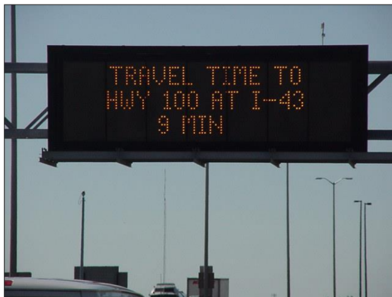
Figure 4.2.3-45: Typical Dynamic Message Sign.
