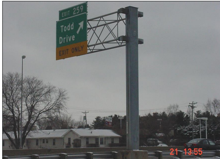
Figure 4.2.3-17: Square Support Column Cantilever (Condition State 1).
