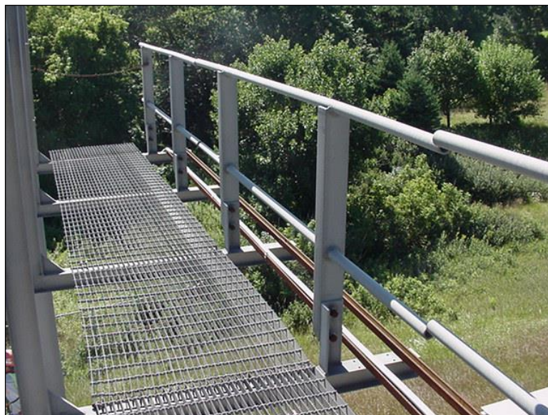
Figure 4.2.4-8: Catwalk with Handrails in Upright Position.
