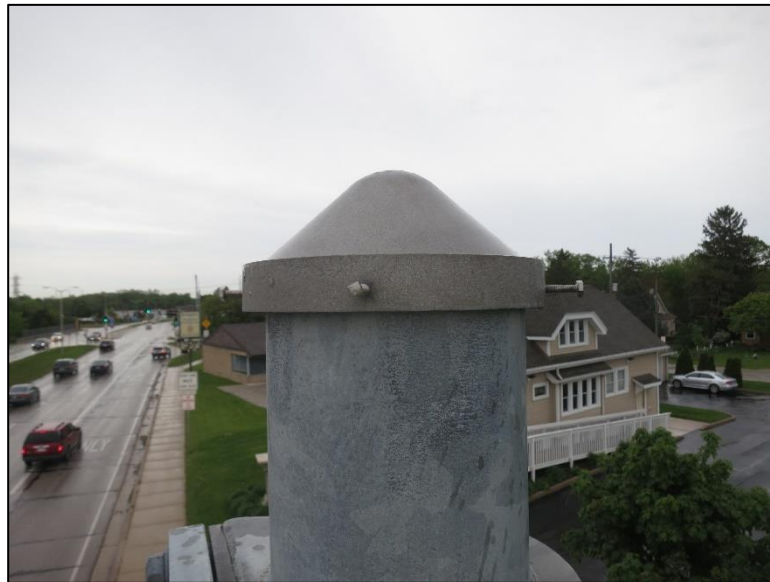
Figure 4.2.4-6: Column Cap for a Two-Chord Sign Structure.
