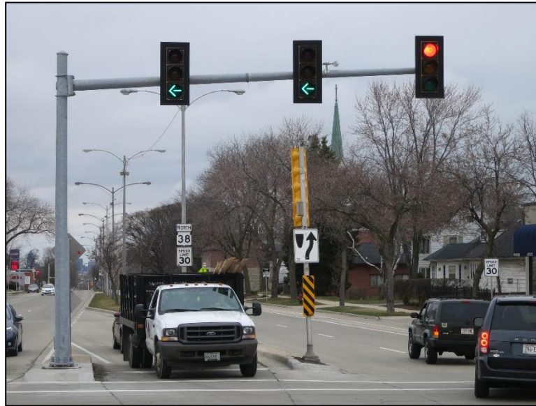
Figure 4.2.3-47: Signal Mast Arm with Three Properly Functioning Signal Heads.
