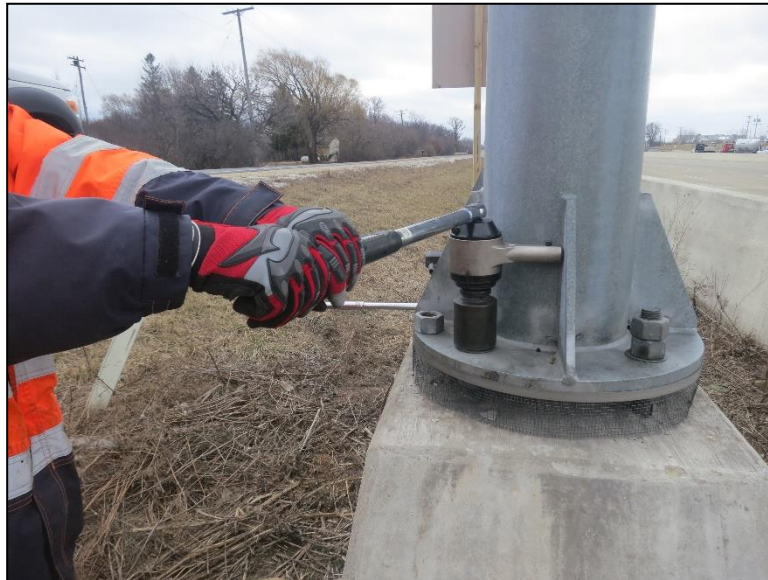
Figure 4.2.3-9: Inspector Using Torque Multiplier to Verify Anchor Rod Tension.
