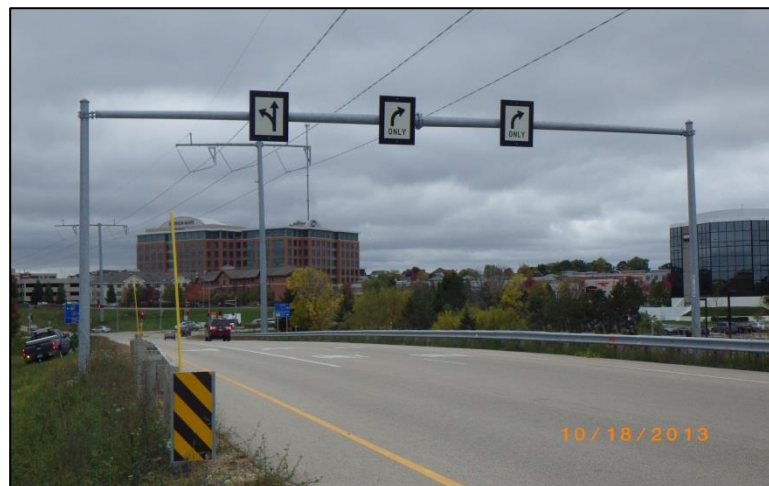
Figure 4.2.1-5: Typical Monotube Sign Support Structure.
