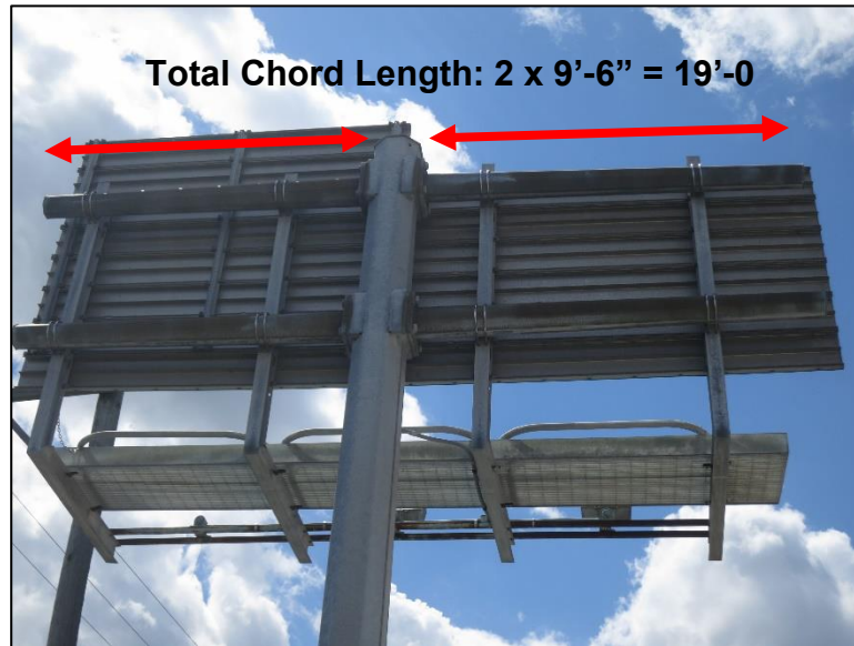
Figure 4.2.3-20: Butterfly Chords Without Trussing.
