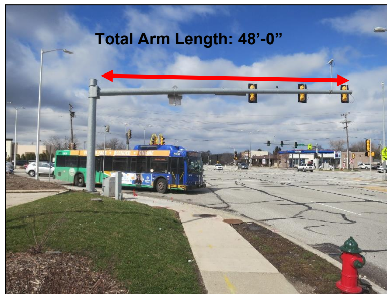
Figure 4.2.3-21: Signal Mast Arm Length.
