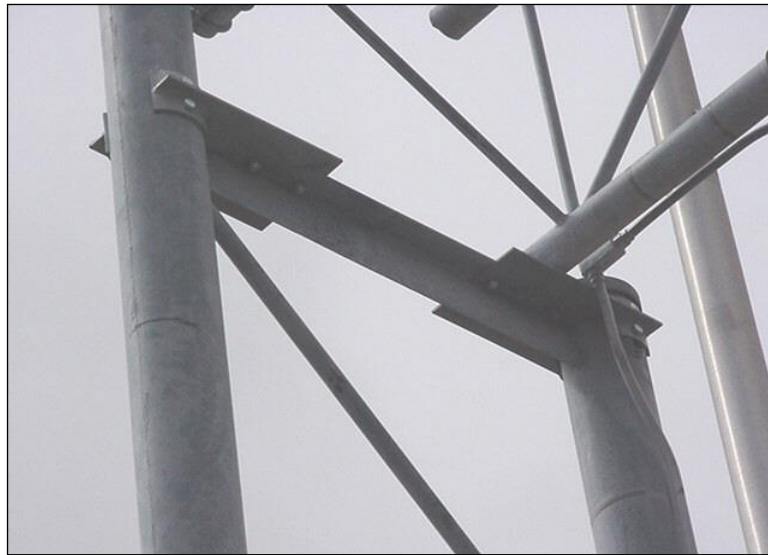
Figure 4.2.3-27: Tri-Chord Bolted T-Section Repair.
