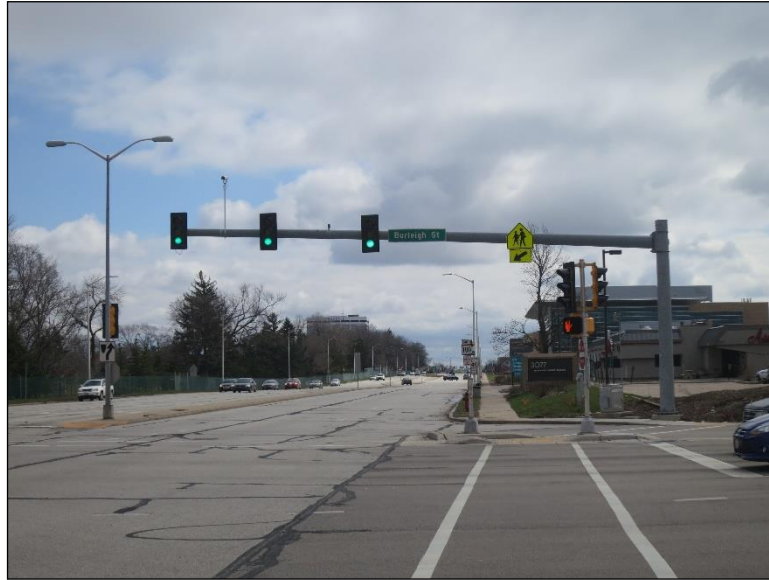
Figure 4.2.1-12: Typical Type 12 Traffic Signal Mast Arm Structure.
