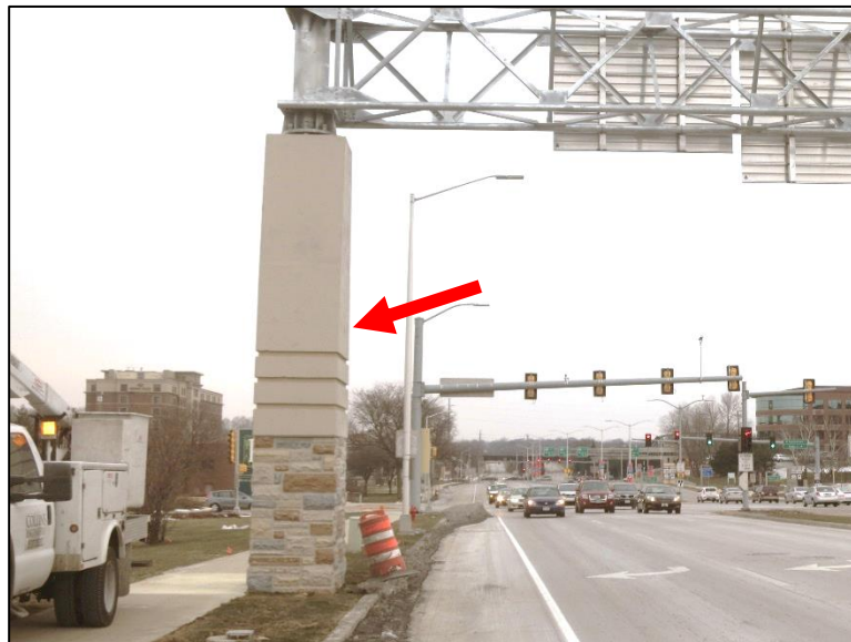
Figure 4.2.4-1: Concrete Pedestal Supporting Four-Chord Cantilever with Form Lined and Stained Concrete.
