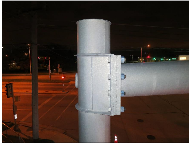
Figure 4.2.3-32: Column to Arm Connection with 8 Bolts. Note Horizontal and Vertical Plates Welded to Vertical Plate.
