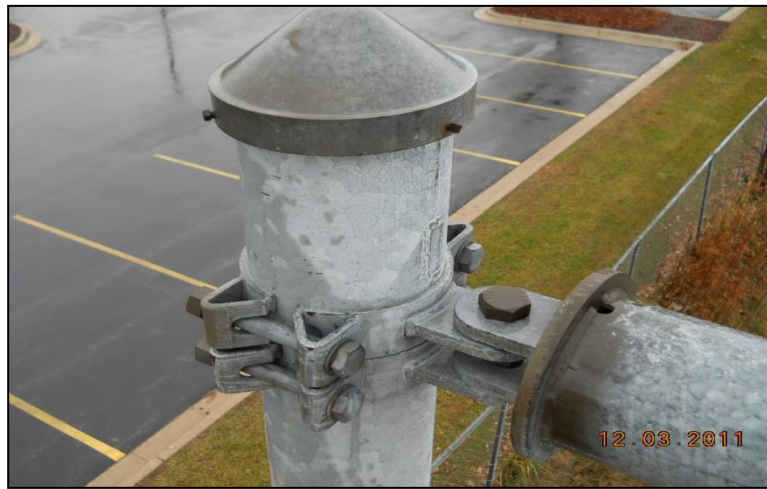
Figure 4.2.3-29: Typical Monotube Chord to Support Column Connection.
