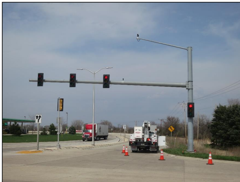
Figure 4.2.1-13: Typical Type 13 Traffic Signal Mast Arm Structure.
