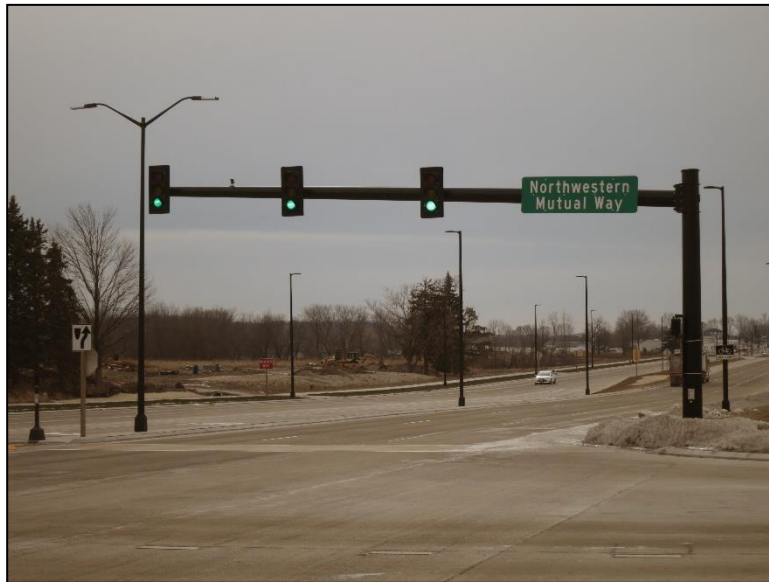
Figure 4.2.4-14: Painted Coating on a Steel Signal Mast Arm Structure (Condition State 1).
