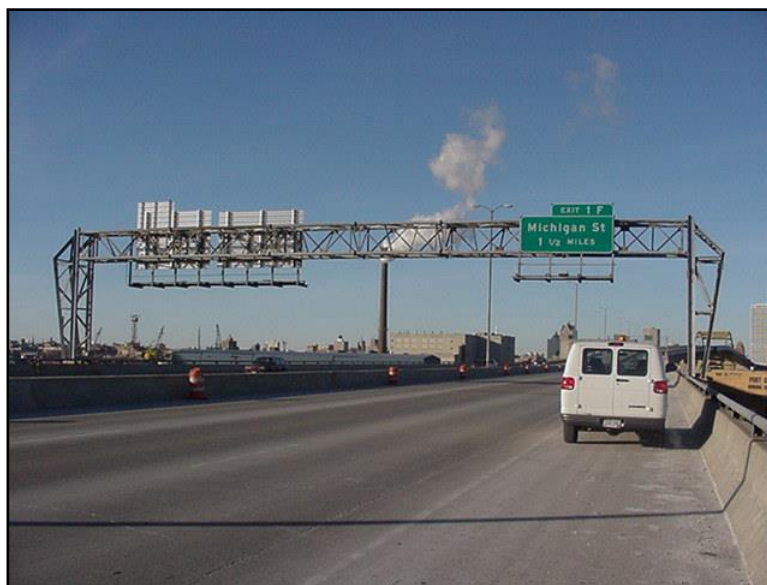
Figure 4.2.1-2: Modified Galvanized Steel Sign Bridge Structure.
