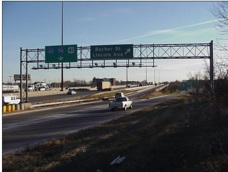
Figure 4.2.1-1: Typical Four-Chord Aluminum Sign Bridge Structure.
