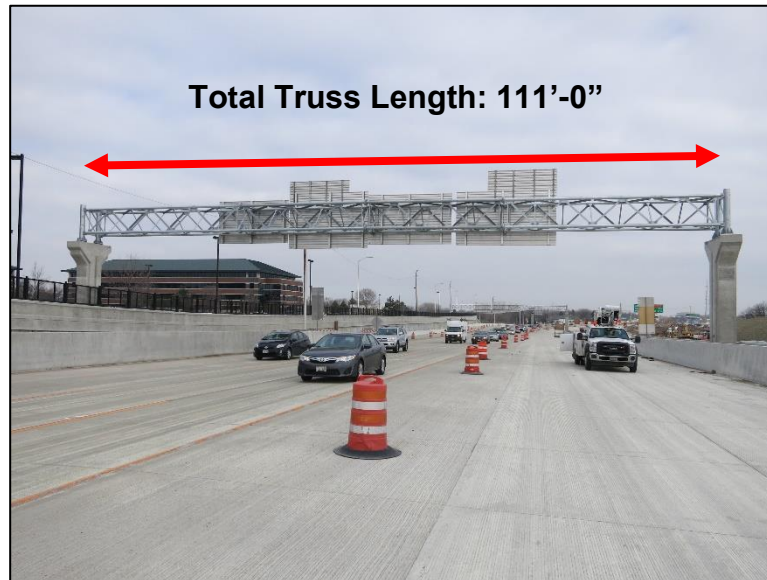
Figure 4.2.3-19: Four Chord Truss.
