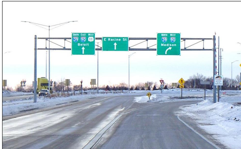
Figure 4.2.1-4: Typical Two-Chord Sign Support Structure.
