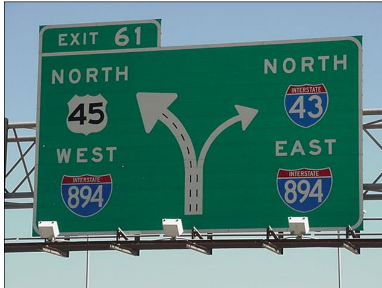
Figure 4.2.3-40: Typical Type I Reflective Sign Panel.
