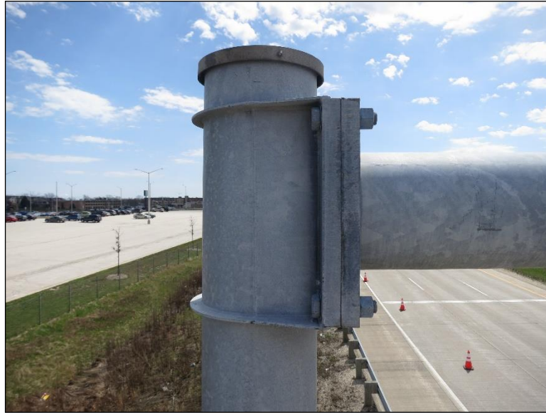
Figure 4.2.1-10: Typical Mast Arm Support Post Connection.
