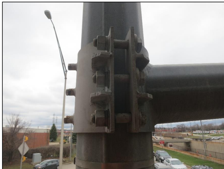
Figure 4.2.3-33: Column to Mast Arm Clamped Connection.
