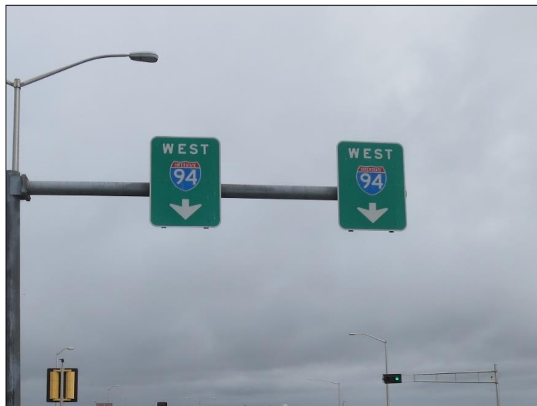
Figure 4.2.3-41: Typical Type II Reflective Sign Panel.
