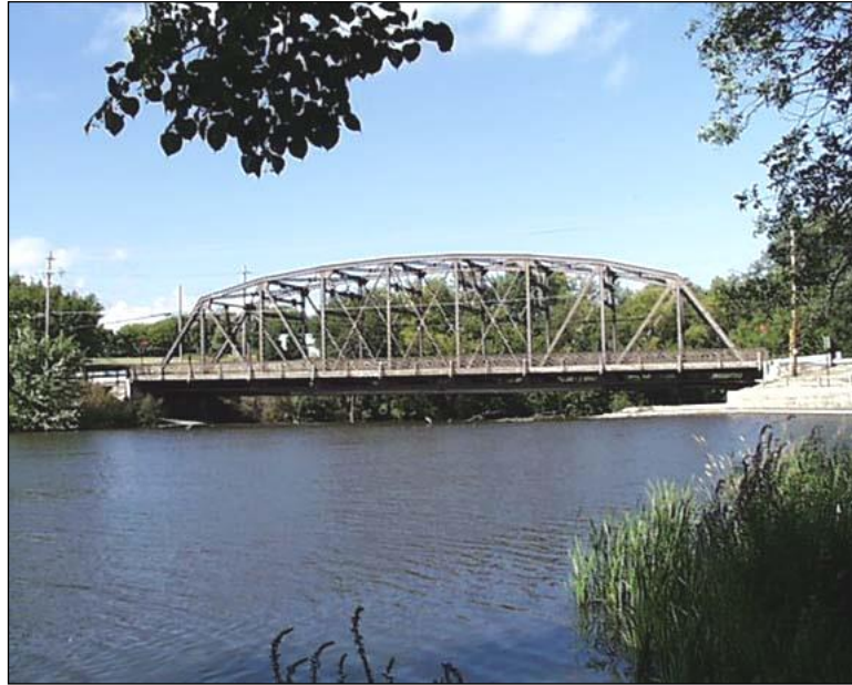
Figure 2.1.5.3-1: Parker Truss Bridge.
