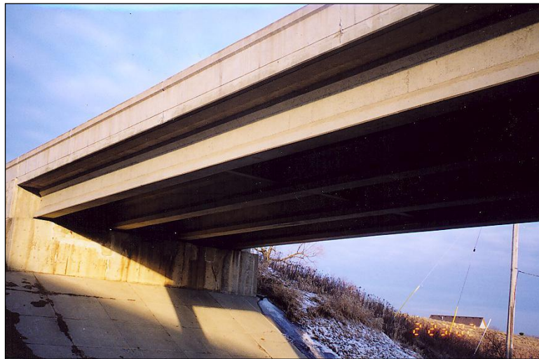
Figure 2.1.5.2-2: Prestressed Concrete Multiple Girder Bridge.
