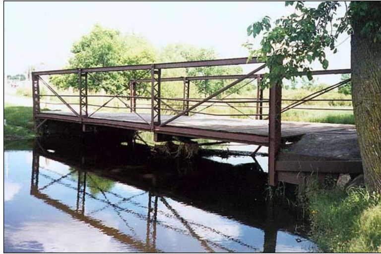
Figure 2.1.5.3-3: Pratt Truss Bridge.
