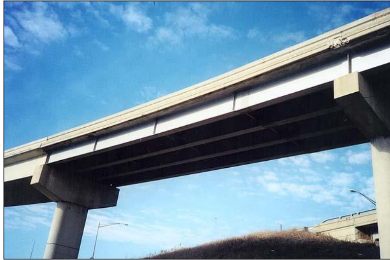
Figure 2.1.5.2-1: Steel Multiple Girder Bridge.
