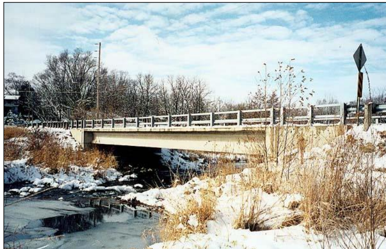
Figure 2.1.2.2-1: Simply Supported Span – Prestressed Concrete Girders.
