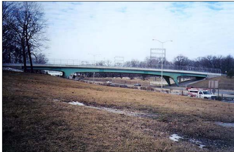
Figure 2.1.5.5-1: Steel Rigid Frame.
