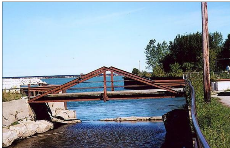
Figure 2.1.5.3-2: King Post Truss Bridge.
