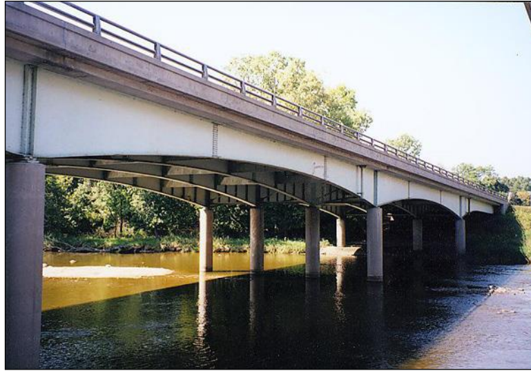
Figure 2.1.2.3-1: Continuous Spans – Steel Girders.
