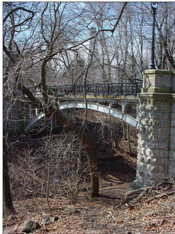
Figure 2.1.5.4-2: Steel Open Spandrel Arch.
