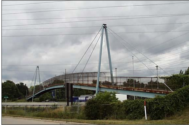
Figure 2.1.5.6-1: Cable-Stayed Pedestrian Bridge.
