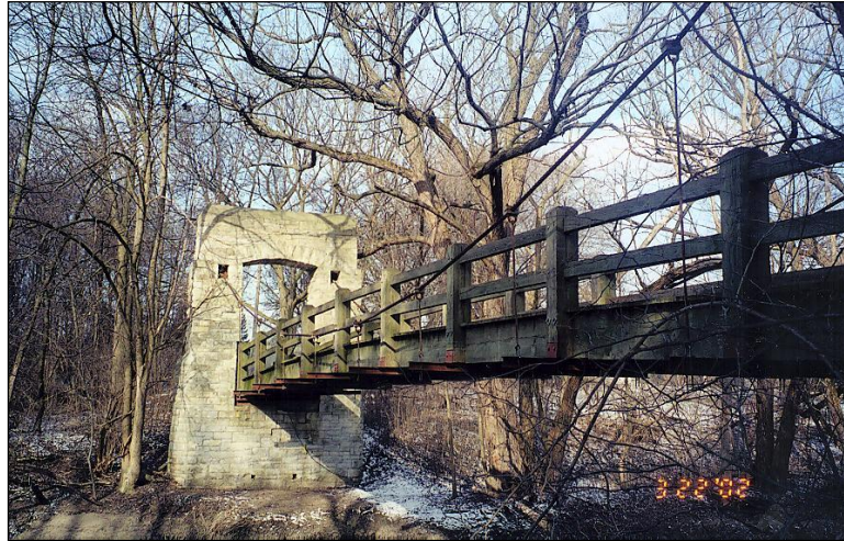
Figure 2.1.5.7-1: Pedestrian Suspension Bridge.
