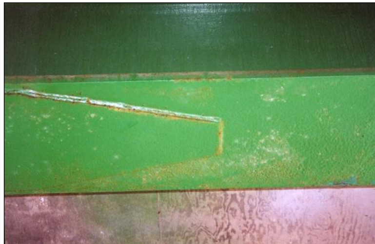
Figure 2.1.4.2-2: Transverse Weld at a Cover Plate End.
