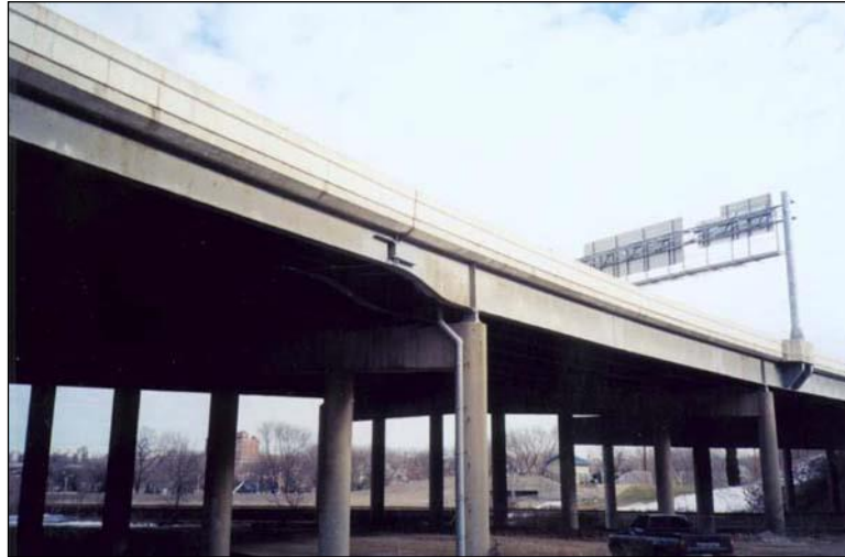
Figure 2.1.2.4-1: Steel Cantilever Span.
