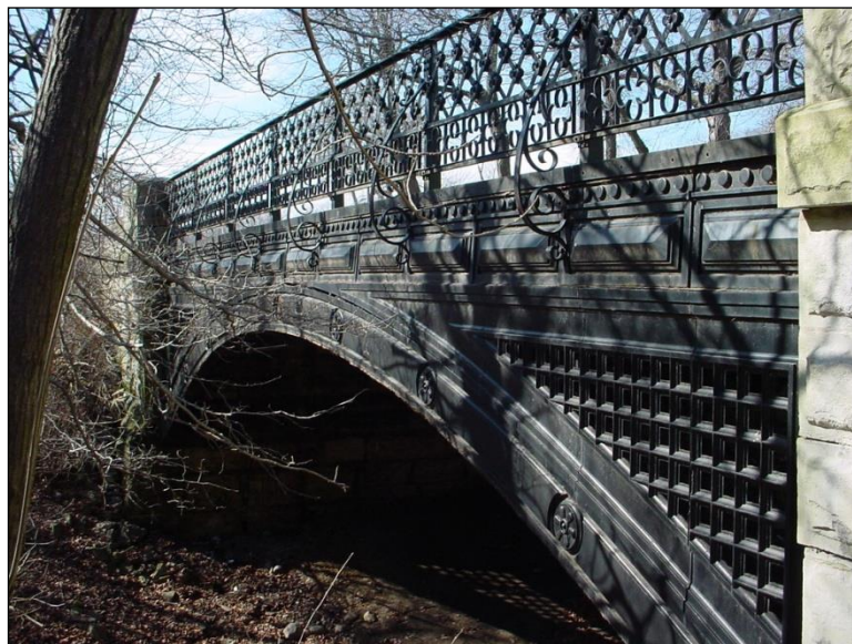
Figure 2.1.4.4-3: Cast Iron Arch.
