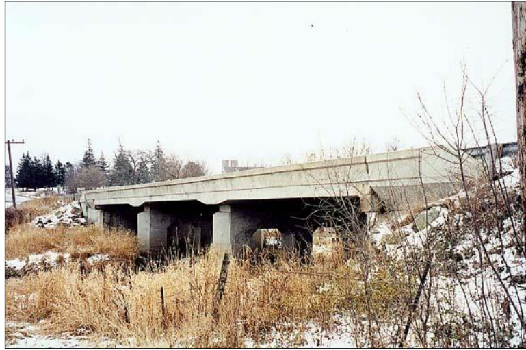
Figure 2.1.5.1-2: Three-Span Concrete Slab with Haunches.
