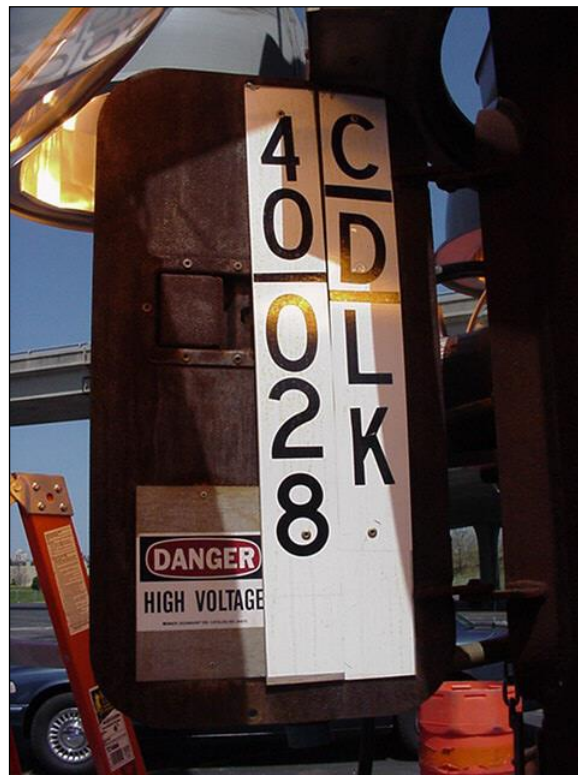
Figure 1.5.2.3-1: Structure Plaque and Circuit Plaque Mounted on a High mast Hatch Door. (Note that the location number “028” would read “0028” according to current convention.)
