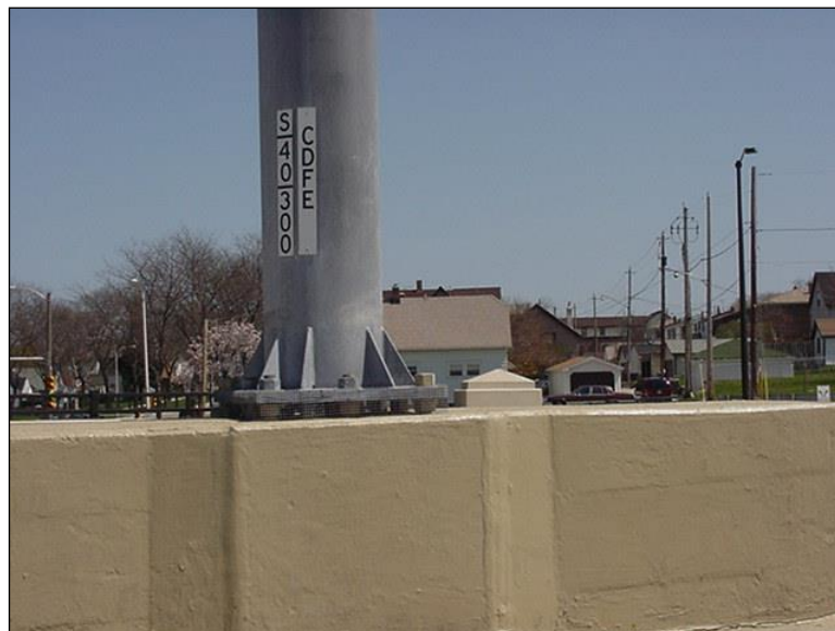
Figure 1.5.2.2-1: Structure Plaque and Circuit Plaque Mounted on a Sign Bridge. (Note that the location number “300” would read “0300” according to current convention.)
