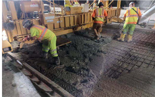
Placement of overlay using double vibrating screed.
