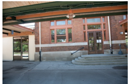
Accessible entrance to building from platforms (on left)
