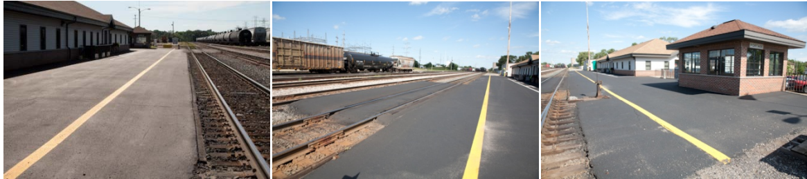
Platform: Below top of rail. Recently resurfaced.
