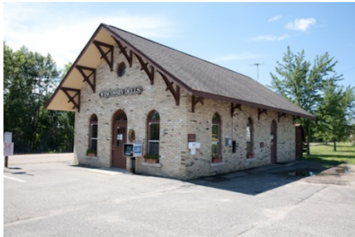
Station building exterior
