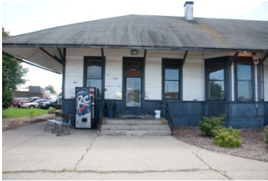
Building, non-accessible entrance to waiting area, vending
