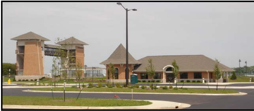
Sturtevant station: View of parking lot, driveway, front of station building, enclosed pedestrian bridge access to platforms, and platform canopy.
