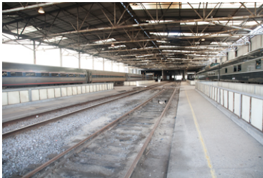
Train shed: platform (non-ADA compliant due to width near tunnel)
