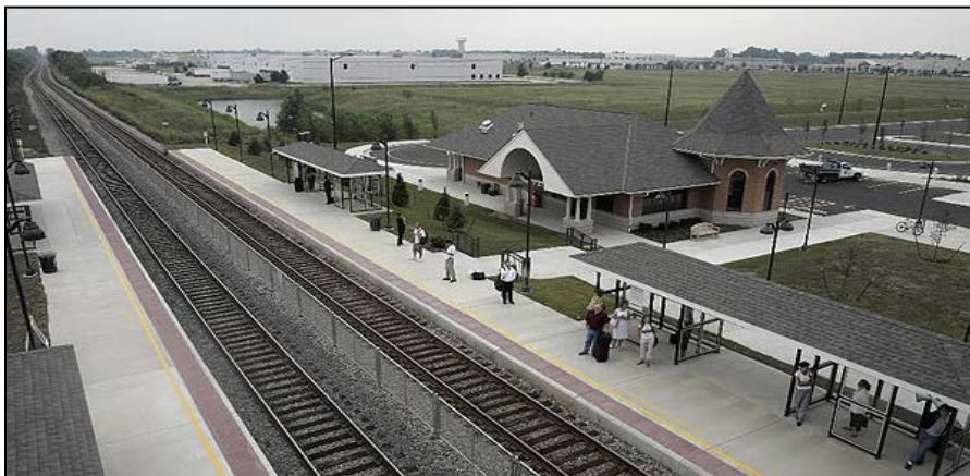
Sturtevant station: platforms with two platform canopies/shelters on each platform; safety fence between tracks.
