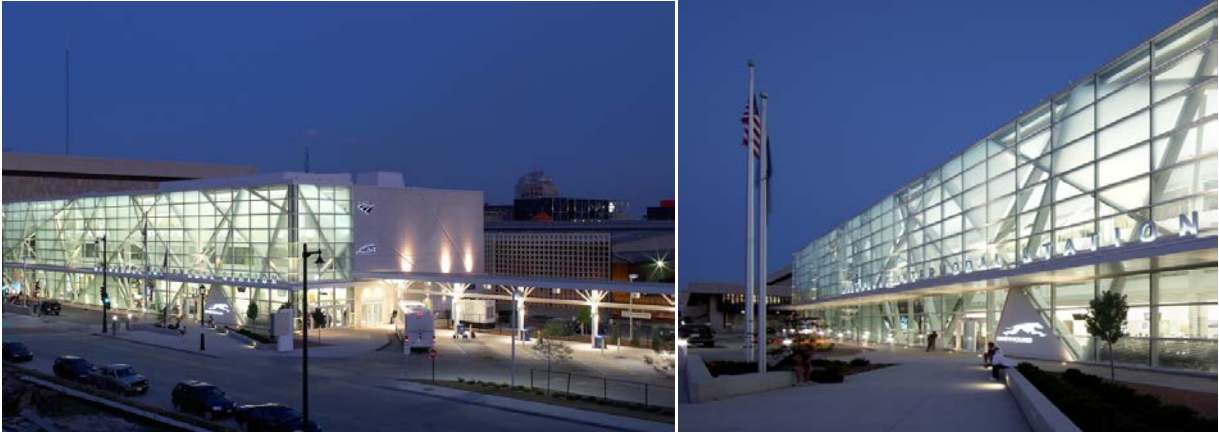
Milwaukee Intermodal Station: building, bus bays for intercity buses, drop-off area, and pedestrian access.
