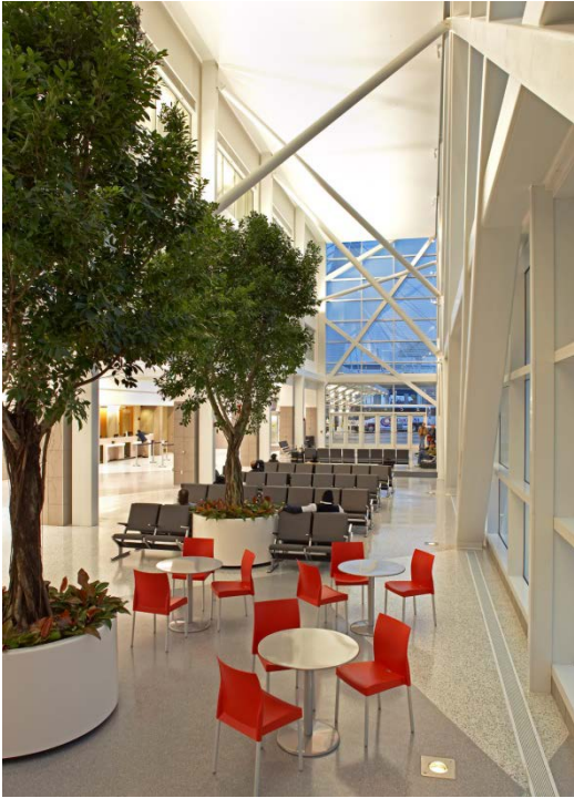
Milwaukee Intermodal Station: interior Amtrak and bus waiting areas.
