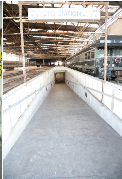
Ramps between platforms and tunnels: non-ADA compliant. Broken concrete and poor condition of tunnel.
