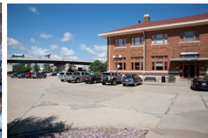
Parking (note cracked concrete and no striping)
