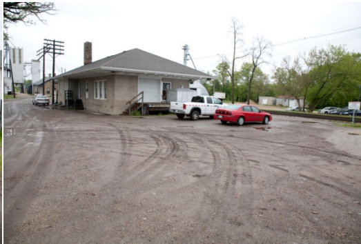
Columbus rail station: entry driveway to station and parking
