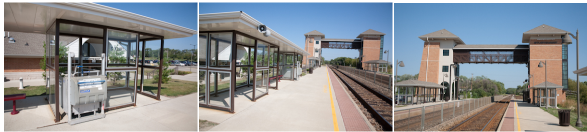
Sturtevant station: Platforms with shelters, wheelchair lift, tactile strip on edge, lighting, access bridge and towers.
