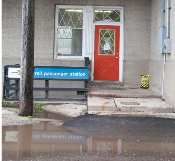
Columbus rail station: entrance to building from driveway and parking (note steps, non-accessible door (narrow, not automatic), and drainage problem).
