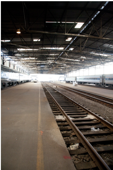
View of one of the below-top-of-rail platforms
