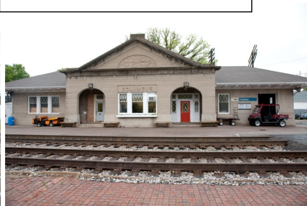
Columbus rail station: view of station from opposite platform (below top of rail, uneven surface, no tactile strip on edge)
