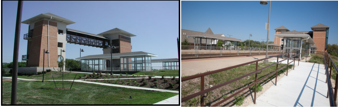
Sturtevant station: pedestrian access to platforms and pedestrian bridge. Platform canopies/shelters.
