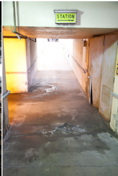
Ramps between platforms and tunnels: non-ADA compliant. Broken concrete and poor condition of tunnel.
