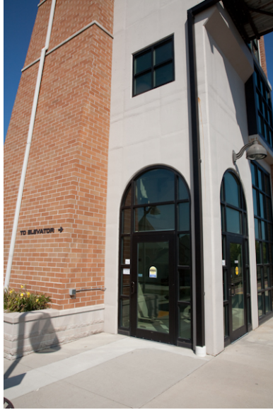
Sturtevant station: Accessible entrance to elevator and pedestrian bridge to platforms.
