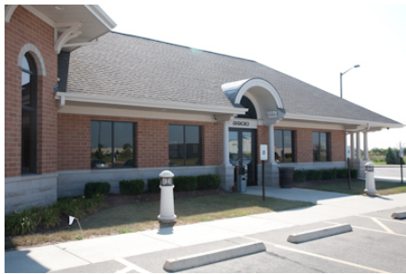
Accessible parking stalls and accessible entrance
