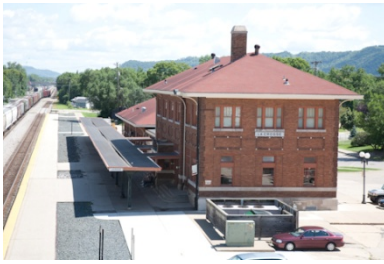
Building and platform and canopy. Note large area between building and platform with ballast.
