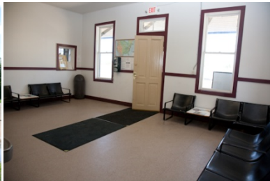
Interior of waiting room. Door not accessible.
