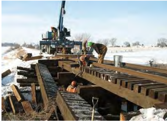
Figure 3-2: WSOR Tie Replacement Photo courtesy of WSOR
