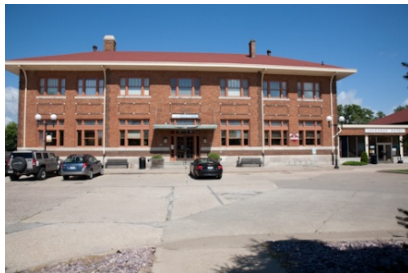
Front of building and parking
