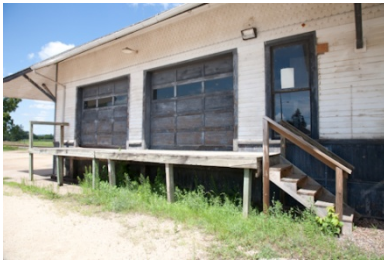
Front of building (from parking/drop off area)
