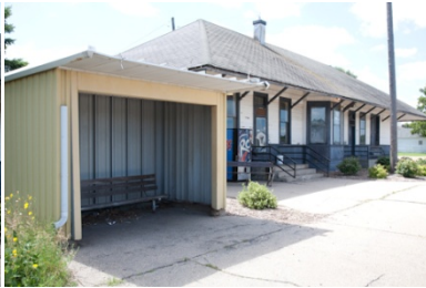
Shelter on platform.
