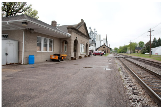
Columbus rail station: platform next to building (below top of rail, no tactile strip on edge)
