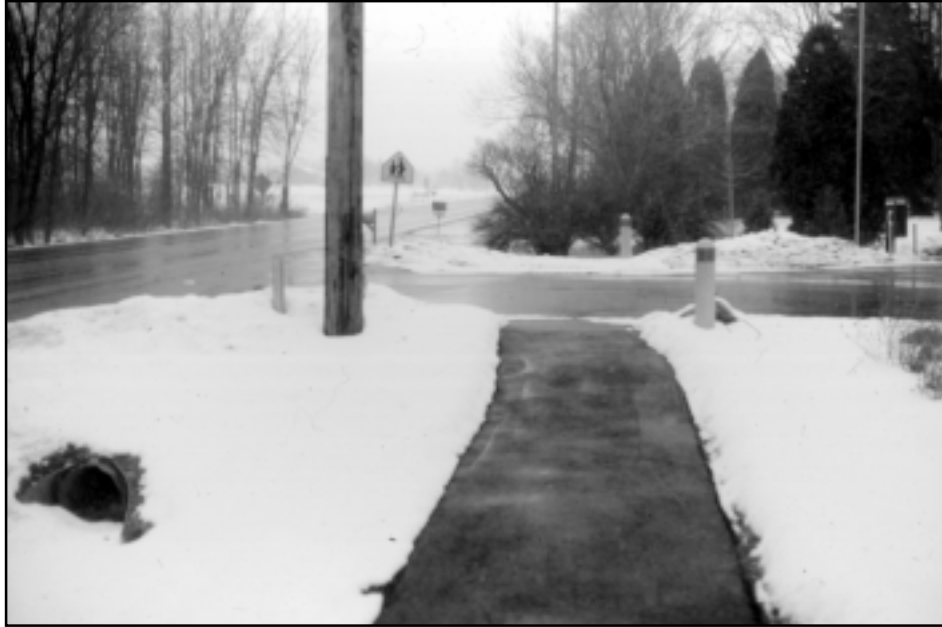
Figure V.3: Local policies concerning snow removal are one important aspect of safe pedestrian facilities
