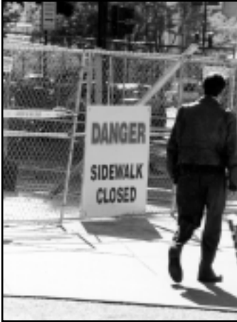
Figure IV.5: When a sidewalk is under construction, alternative facilities marked appropriately become critical for blind pedestrians who are unable to read signs by sight
