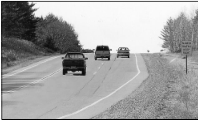
Figure 33. Passing lanes can be an effective strategy to enhance safety on rural two-lane highways.
