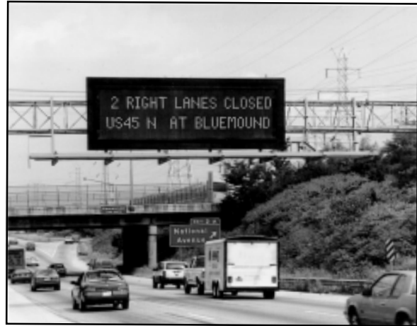
Figure 27. New technologies can improve the flow of traffic by providing travelers with up-to-the-minute road conditions.
