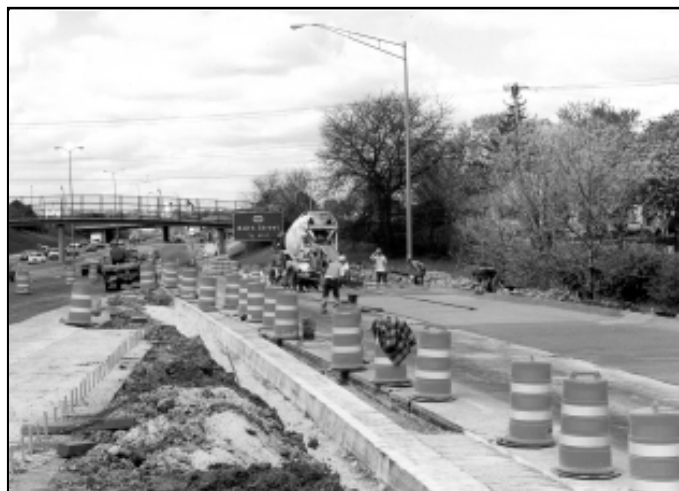
Figure 24. SHP 2020 calls for interchange upgrades to improve capacity and traffic flow.
