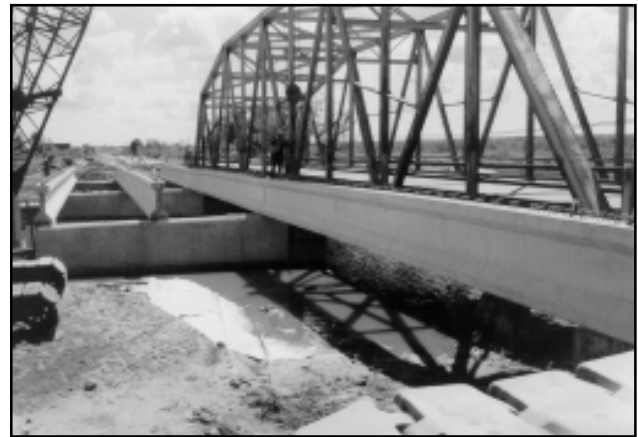
Figure 41. During the next 21 years, WisDOT will replace approximately 335 bridges over water.
