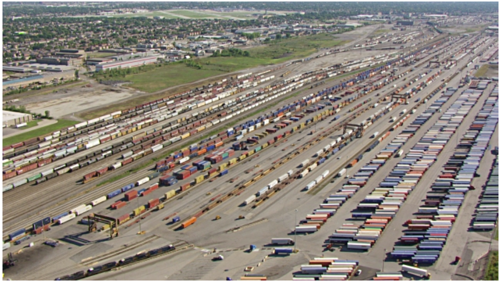
Image 22: CSX Bedford Park Intermodal Terminal (Source: Bright India Group).
