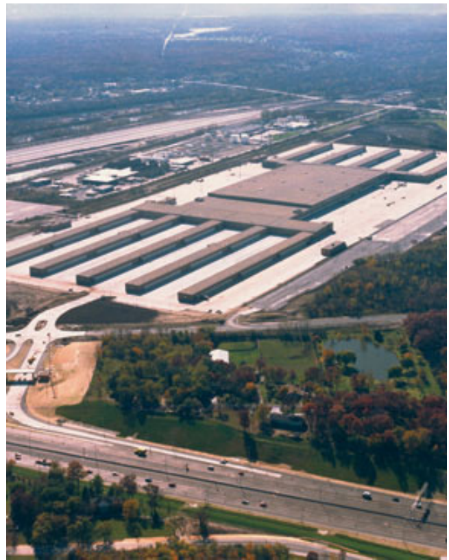
Image 21: UPS CACH Facility, Hodgkins, IL (Source: Power Construction).
