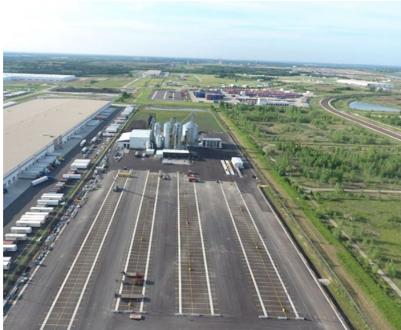
Image 23: The DeLong Co., Inc. Joliet South Container Loading Facility (Source: The DeLong Co., Inc).
