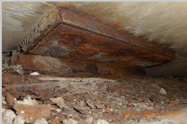
Bearing in shiplap joint no longer aligned with pad
