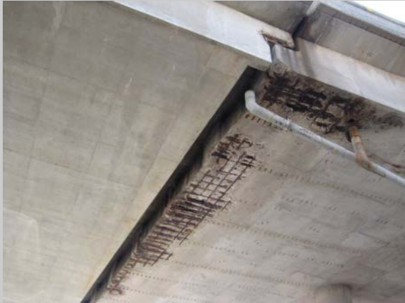
Deterioration at shiplap joint
